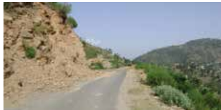
Construction of 9 km (BTR) road from Gali to Kinari
