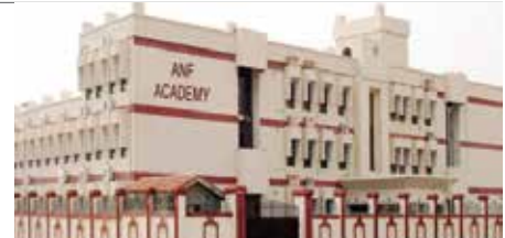
New ANF Academy Building
